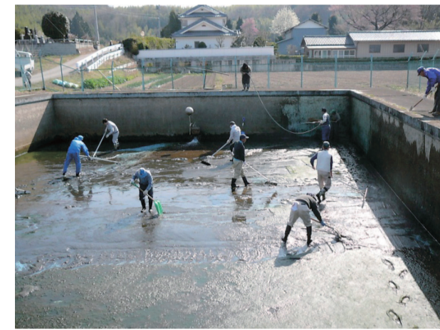
Local residents taking part in cleaning of a regulating pond
